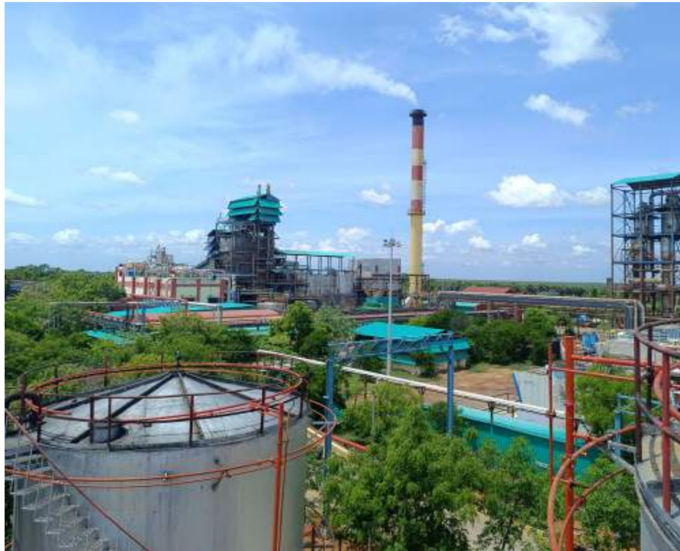
Our standalone distillery plant at Sivaganga
