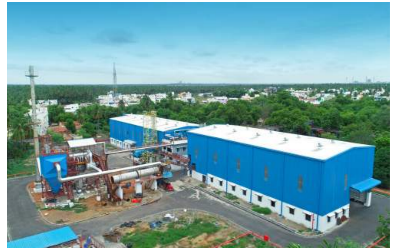
Sugar and Co-generation Plant at Pugalur generating 4800 TCD, 22MW
